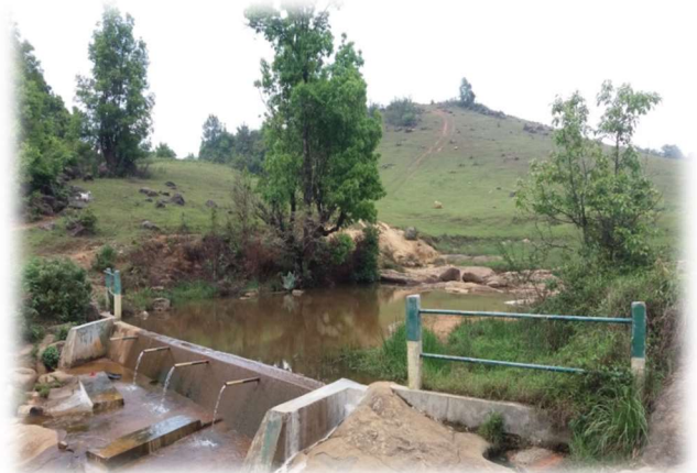
CHECK DAM CUM WASHING PLACE AT THIEPKSEH UNDER UMTYNRU WEISAR WATERSHED
