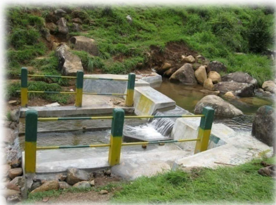
HEAD WATER DAM CUM WASHING PLACE AT SANGRIANG UNDER WEINIER WATERSHED
